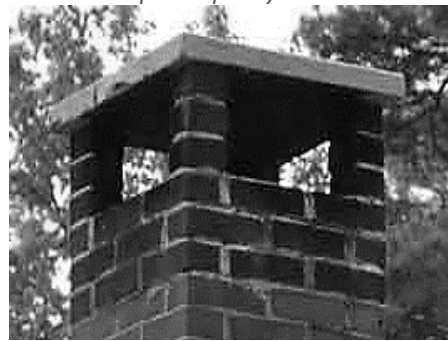
Concrete Cap Chimney Top
