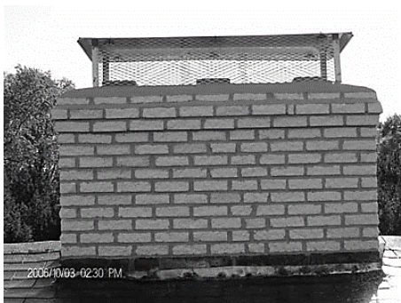
Metal Cap on Clay Liner Chimney Top
