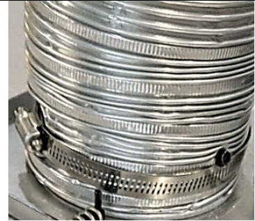
Vent Adapter Flex Connection Hose Clamp first. Secure w/ Screw above Hose Clamp
